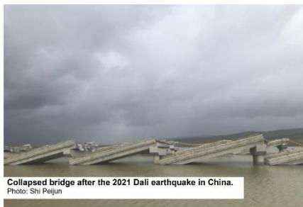
Collapsed bridge after the 2021 Dali earthquake in China.
