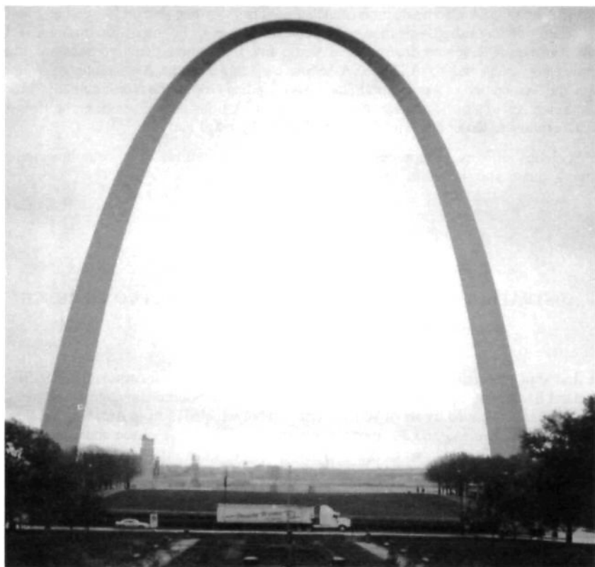
The Gateway Arch, the nation's tallest manmade monument, commemorates St. Louis' vital role as the gateway to the West. The 630' Arch, designed by Architect Eero Saarinen is a classic weighted inverted catenary curve of stainless steel (total weight 43,000 tons), built 1963-65.
